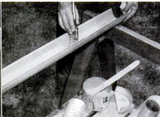
ON GUTTERS AND DOWNSPOUTS before you install them. You can add a top coat of regular paint later to match the color of your house.
