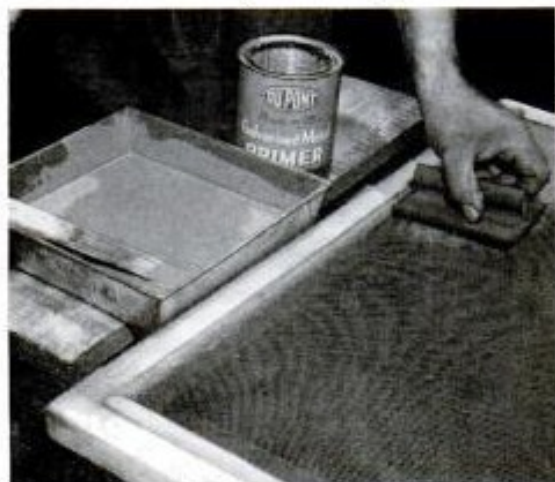
ON GALVANIZED SCREENS to prevent rust; on copper screens to avoid staining on wood frame. Using a scrubber minimizes clogging of mesh.
